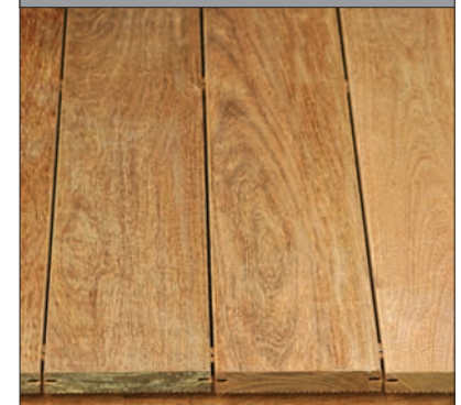
Repeat steps 2 and 3 until the last deck board is installed. Repeat step 1 to attach the last board
