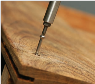
Drill the holes for the plugs - Screw the 1st deck board - Insert the plugs
