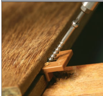
Insert the fastener - Screw the fastener at approximately a 45° angle through the deck board and down into joist
