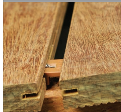
Install the next deck board until it abuts the integrated spacer
