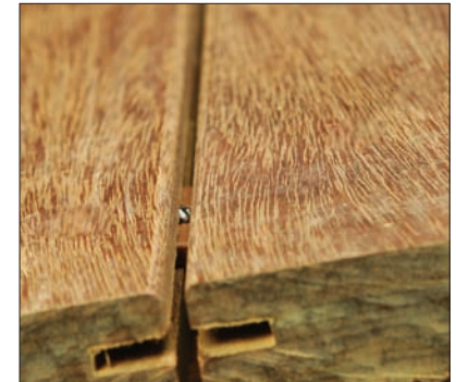
Repeat steps 2 and 3 until the last deck board is installed. Repeat step 1 to attach the last board
