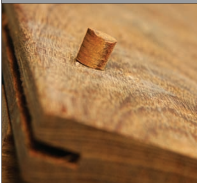
Drill the holes for the plugs - Screw the 1st deck board - Insert the plugs
